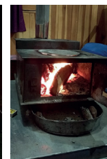
Wood heater with chimney
